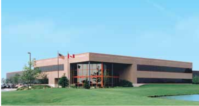
Clockwise from bottom: WaterFurnace International world headquarters. Buckingham Palace utilizes geothermal. A typical geothermal installation.
